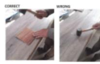
Place a scrap piece of plank over the end joint seam and tap LIGHTLY with a rubber mallet. NEVER strike the planks directly as this may fracture the locking system and eventually cause end joint failure.
